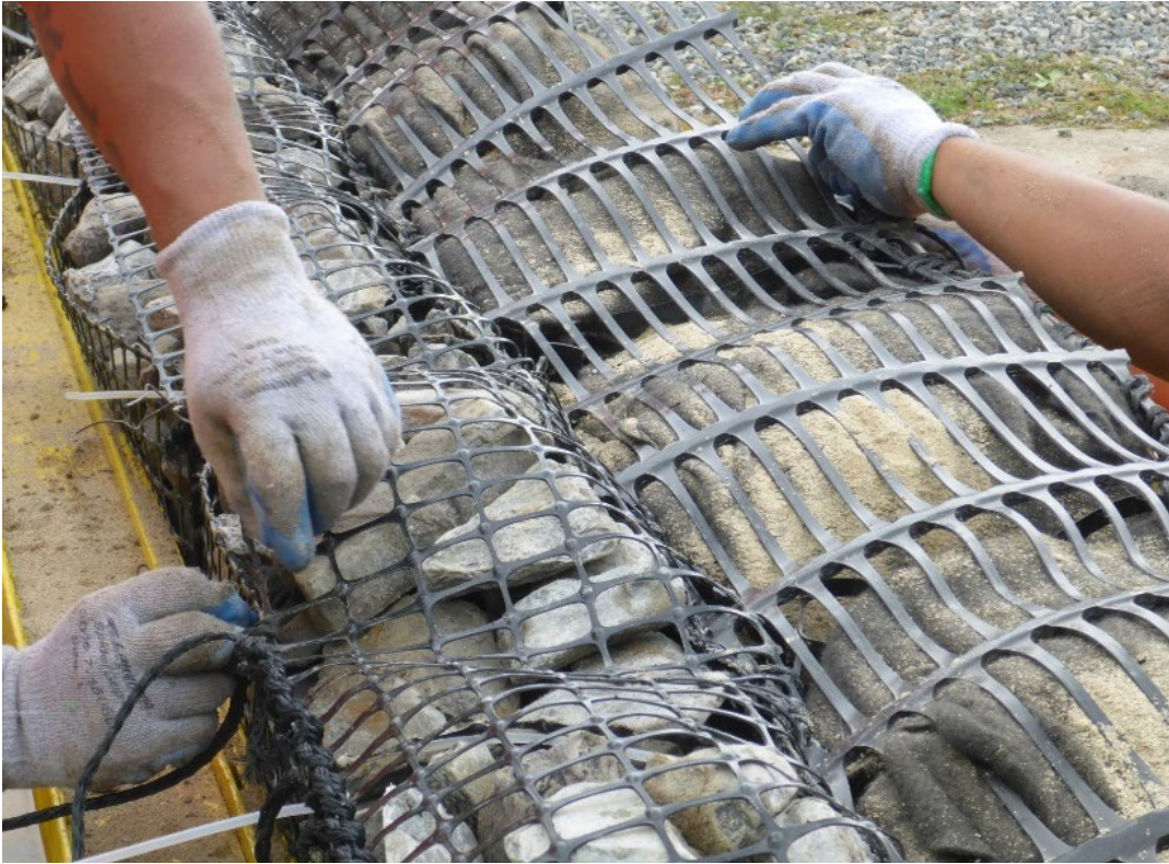
MAM filled with armor material (left) and sand/organoclay in geotextile bag (right)
