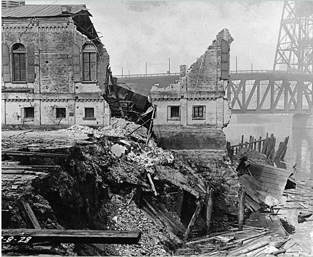
Former PGM plant structure
