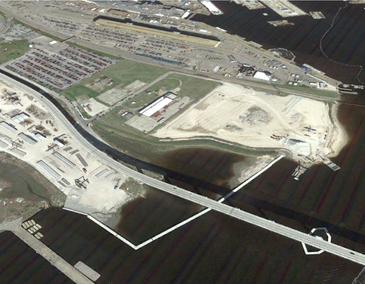
During remedial construction
