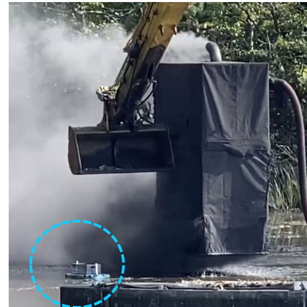
Floating catch pan in swing path
